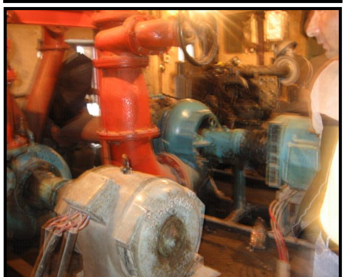
Photo Slides shows pumping station facilities in highly dilapidated condition which was further damaged with recent major floods in Sept 2014
