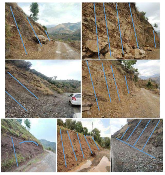
Figure 5.5: Critical Landslip/ erosion sites identified sections having stabilization issues falling in Barot and Gambir Mughlian areas of Gulhati to Shahdra Sharief Road
