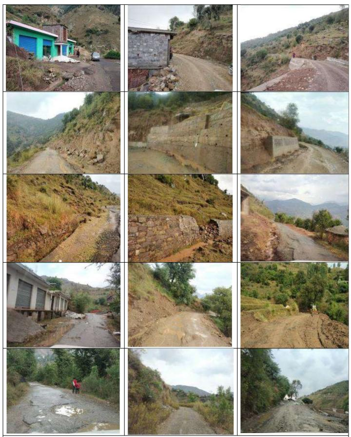
As evident from the site photos, non-existence of hill road drainage road surface is in a degraded state. The exisiting protection walls are old and disintegrating over the period of time and possess potential negative safety issues of the proposed road.
