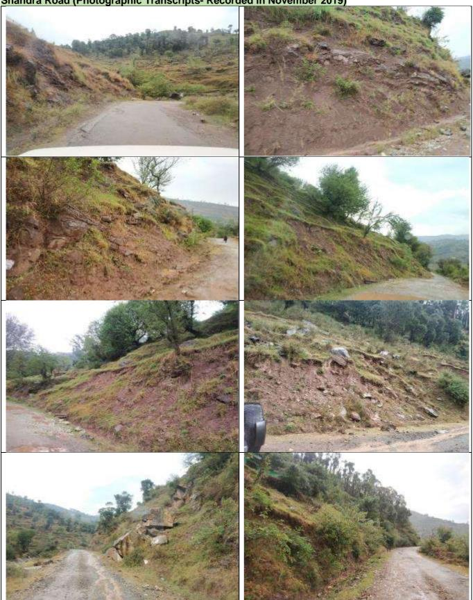
Gulhati to Ghambir Mughlian road showing the sections from 0+300 to 9+500 which require bio-stabilization and protective slope measures
