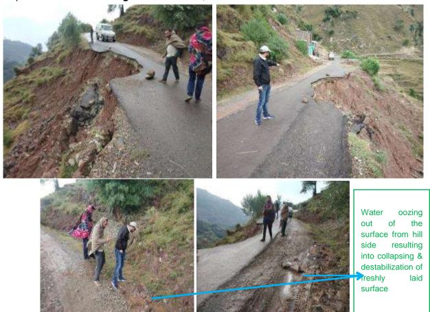
Fig: 5.4: Fresh landslip/erosion case in Ghala area at Ch 12+600.
