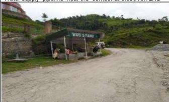
Bus Bay and damaged road surface at Ch 0.050 Km
