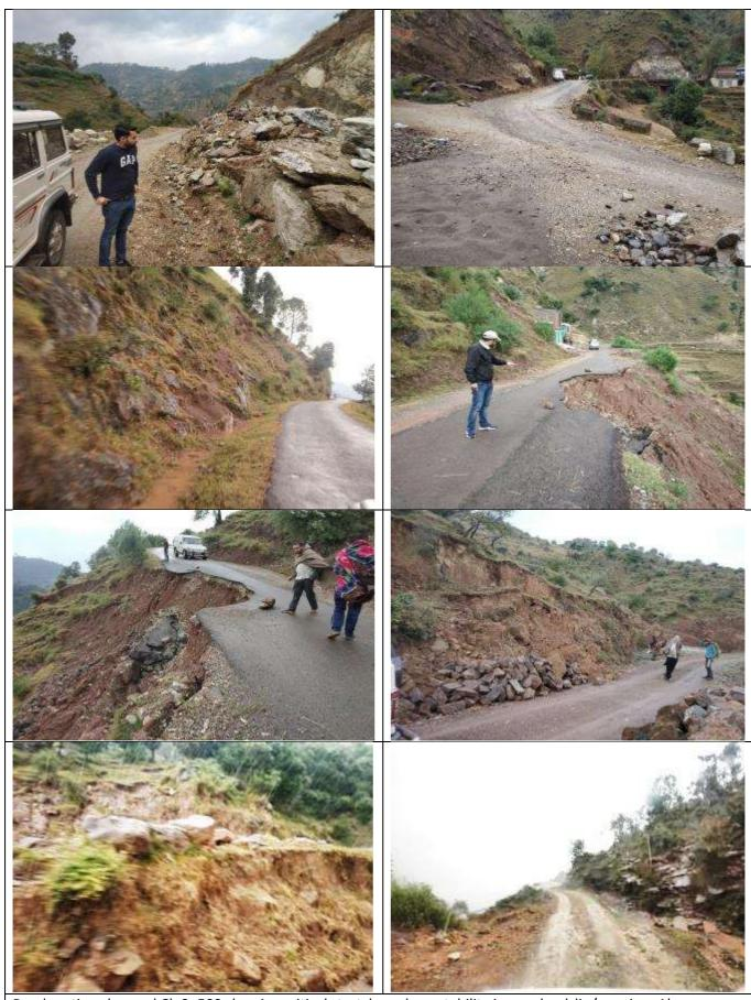
Road sections beyond Ch 9+500 showing critical stretches slope stability issues, landslip/erosion. Above photographs showing stability issues also include Ch 10+000- 15+000 which is already upgraded under PMGSY.
