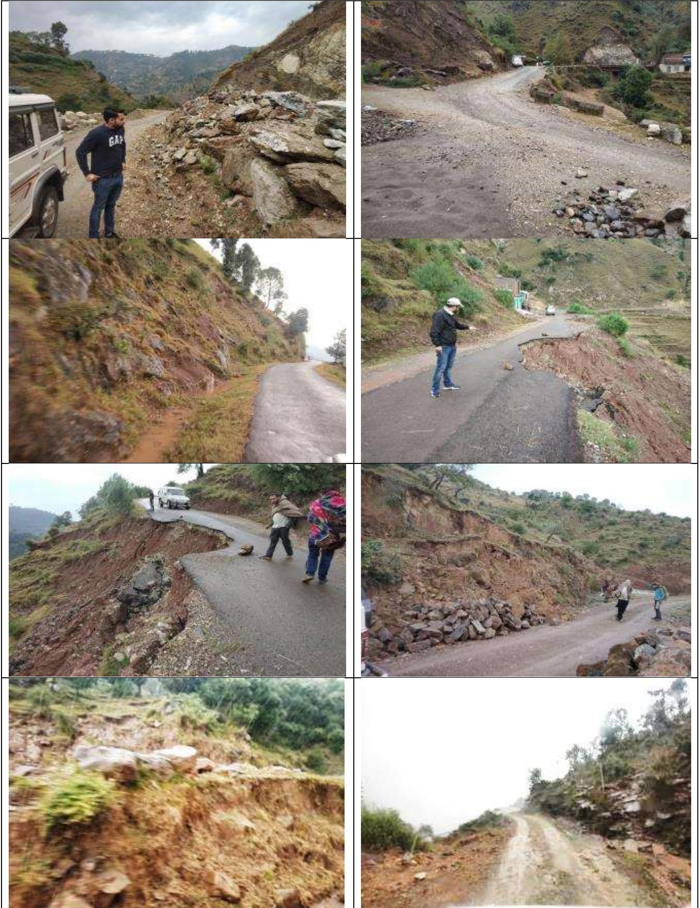
Road sections beyond Ch 9+500 showing critical stretches slope stability issues, landslip/ erosion. Above photographs showing stability issues also include Ch 10+000- 15+000 which is already upgraded under PMGSY.
