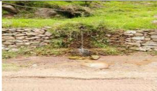
Road getting damaged due to water flowing into the Corridor at Ch 2.500 Km RHS
