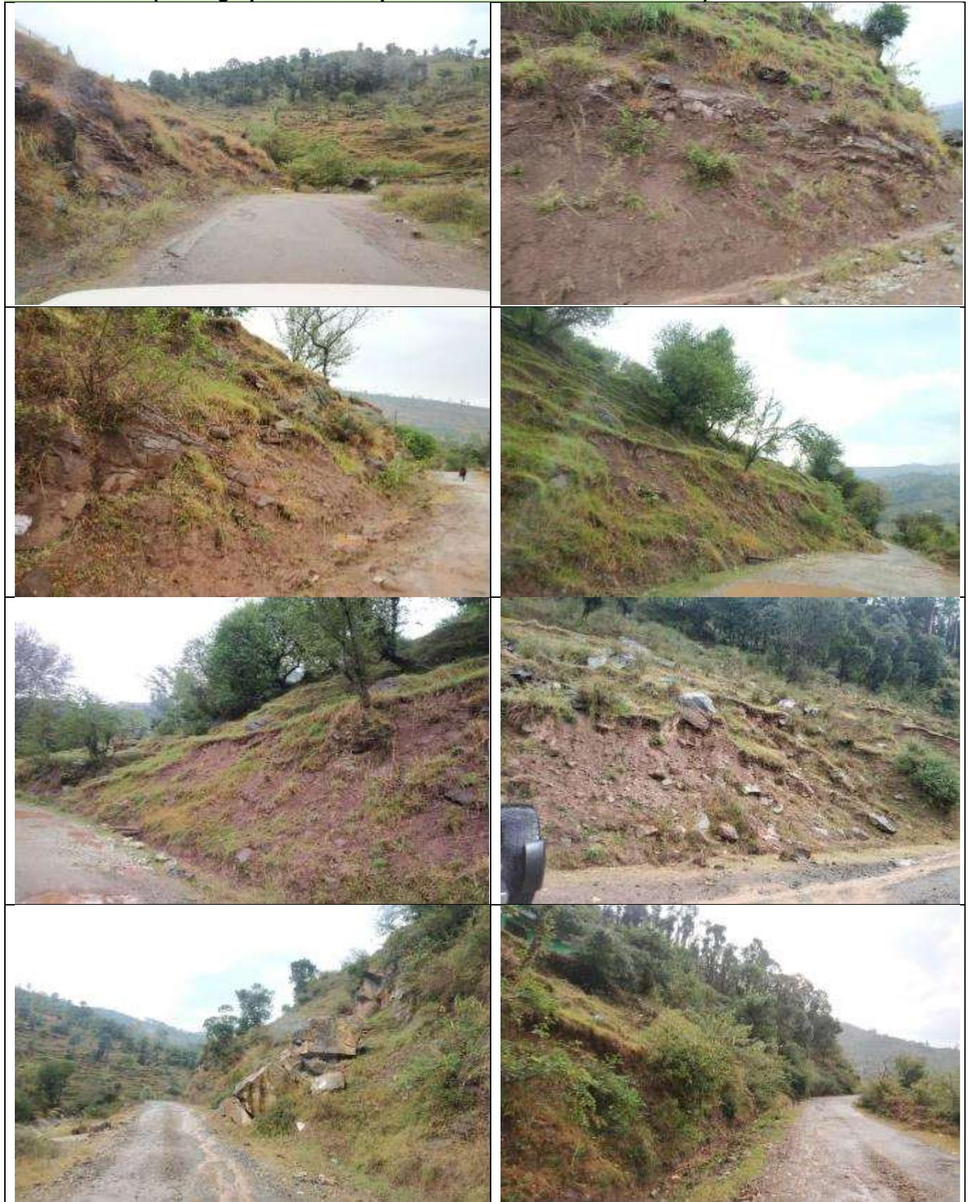
Gulhati to Ghambir Mughlian road showing the sections from 0+300 to 9+500 which require bio-stabilization and protective slope measures
